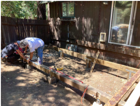
Building a new deck for the Maintenance Cabin
